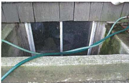
Foundation level of the Caretaker's Cottage, showing non-original windows, which can be replaced
