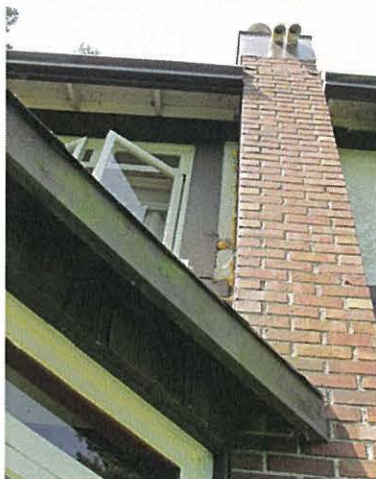
One of the exterior chimneys on rear of house
