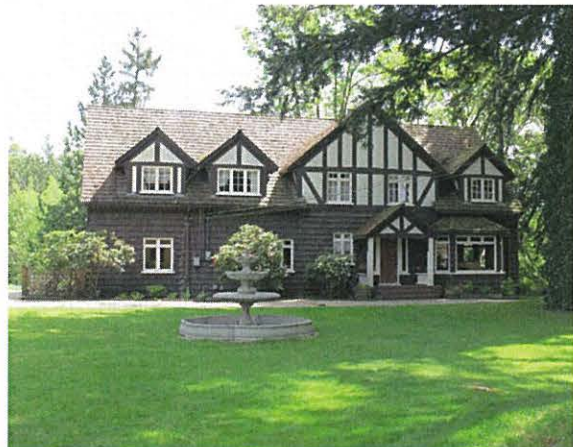
Main roof structure
