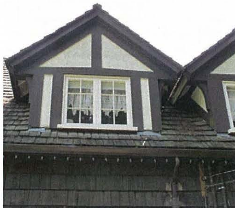
Original windows of the front façade
