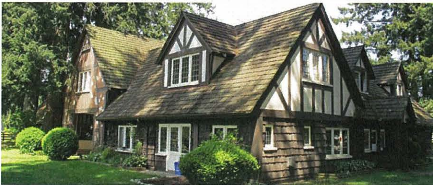
Original windows on the south and east elevations
