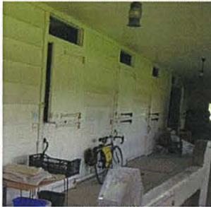
North elevation former stable doors
