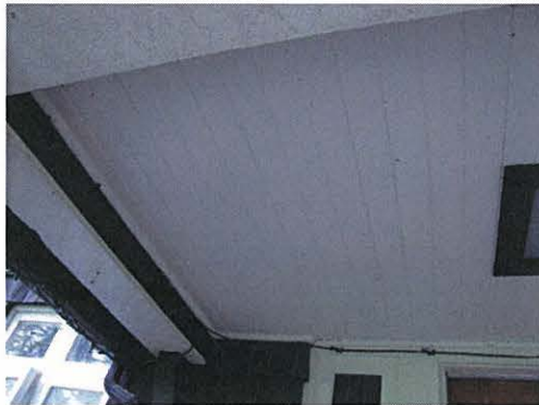
Closed soffits, main entry
