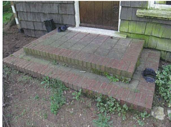
North elevation: brick steps
