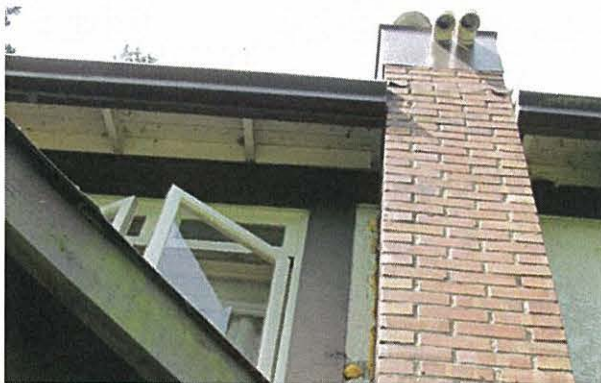
Open soffits and exposed rafter tails
