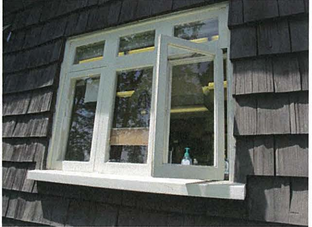
Additional original window assemblies – note the presence of tripartite assemblies as well as single windows with multi-paned transoms
