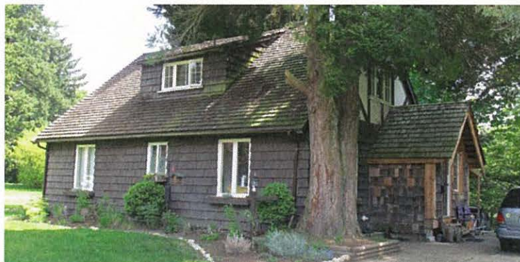
West elevation: gabled main roof and shed roof dormer
