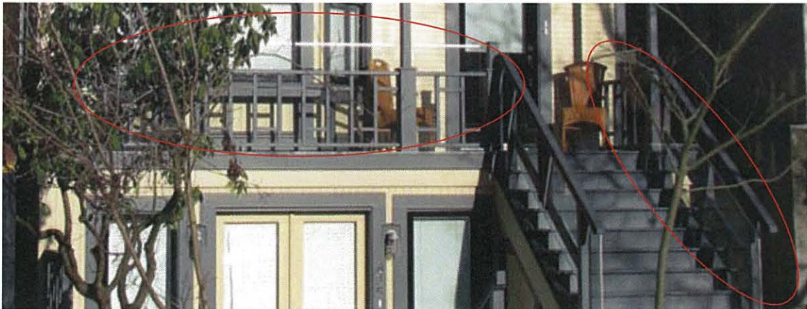
Code compliant balustrade, circled in red; the glass inserts are barely visible. A metal handrail installed on the staircase would also be a reversible and acceptable solution.
