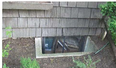
Foundation level of the Caretaker's Cottage, showing non-original windows, which can be replaced
