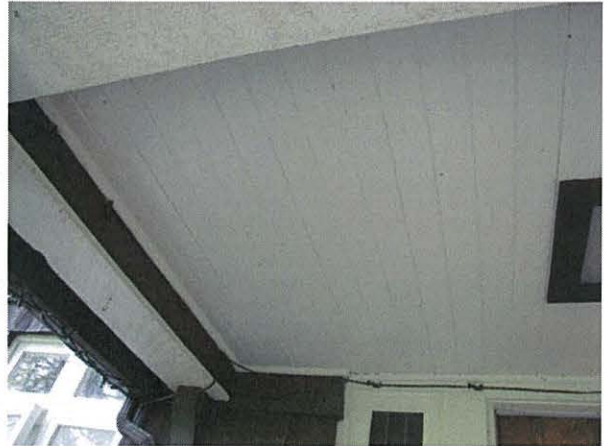
Closed soffit ceiling of front entryway
