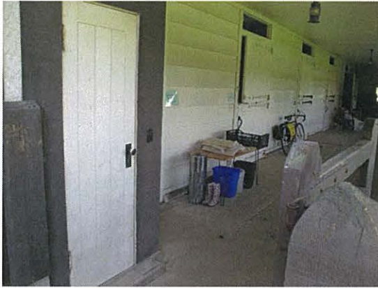
North elevation: wooden lapped siding along former stables
