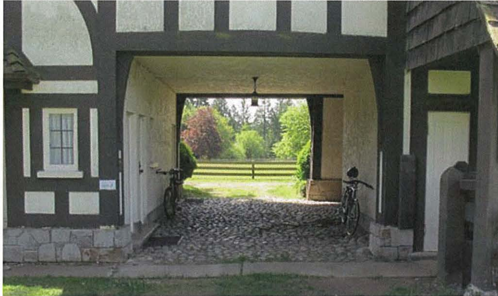
Tunnel, looking south
