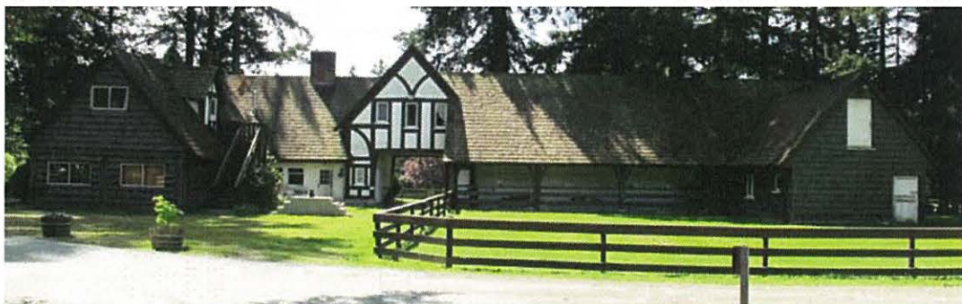
Main roof structure of the Coach House
