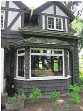
Original windows of the front façade
