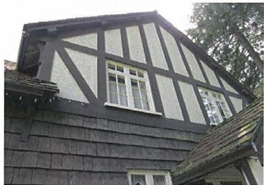
Half-timbering in gable-ends
