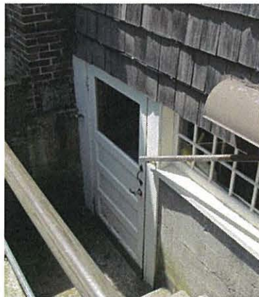
Rear entry door, basement
