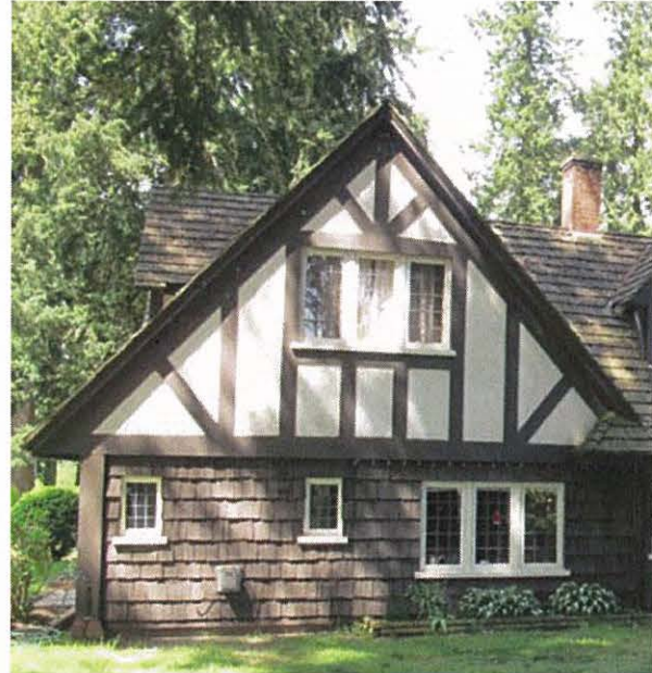
East elevation gable end: cornerboard, bargeboards and projected sills
