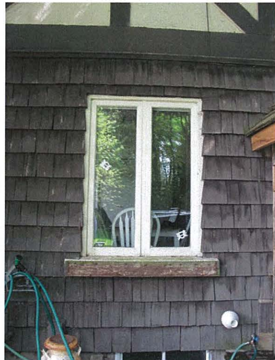
Original window, front façade
