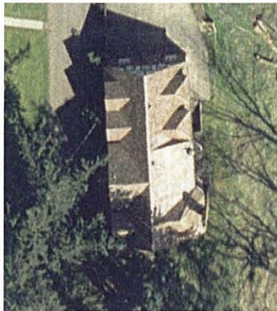
Aerial view of roof structure, Google Maps
