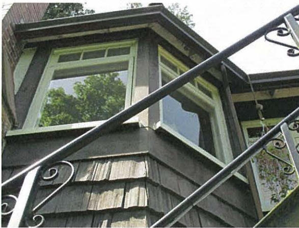
Additional original window assemblies – note the presence of tripartite assemblies as well as single windows with multi-paned transoms
