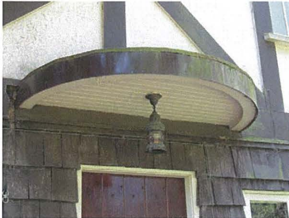
North elevation: semi-circular awning with hanging light fixture
