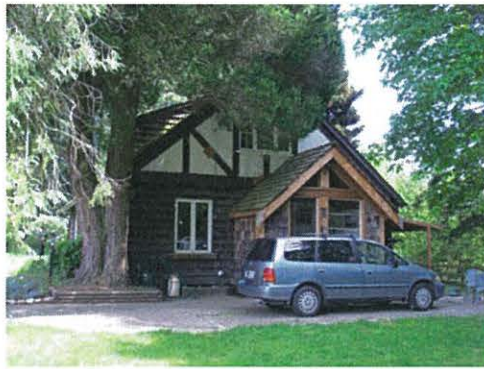
South facade showing existing addition
