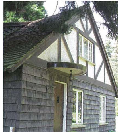
North elevation: bargeboards, half-timbering, wood trim and projected sills
