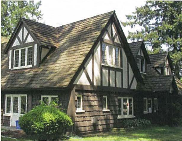
South and east elevation front-gabled dormers
