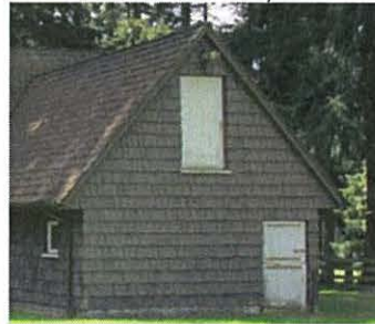
North elevation hay loft and stable doors
