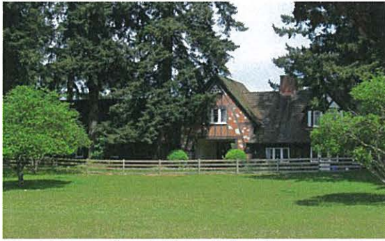
South (front) facade
