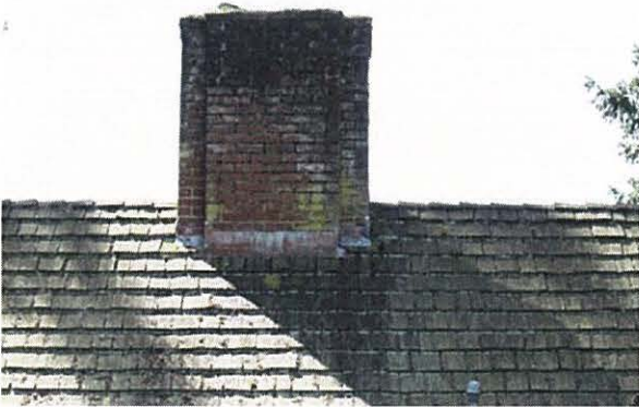
Original interior brick chimney on east-west ridge
