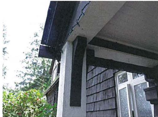
Column and bracket, main entry
