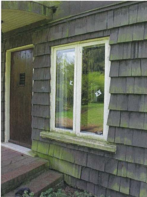
Original windows of the rear façade
