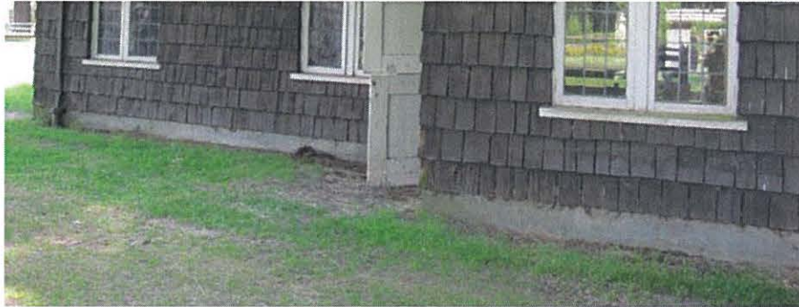
Coach House Foundation (west elevation)
