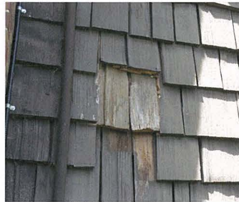
Missing shingles
