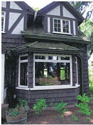
Bay window and dormers
