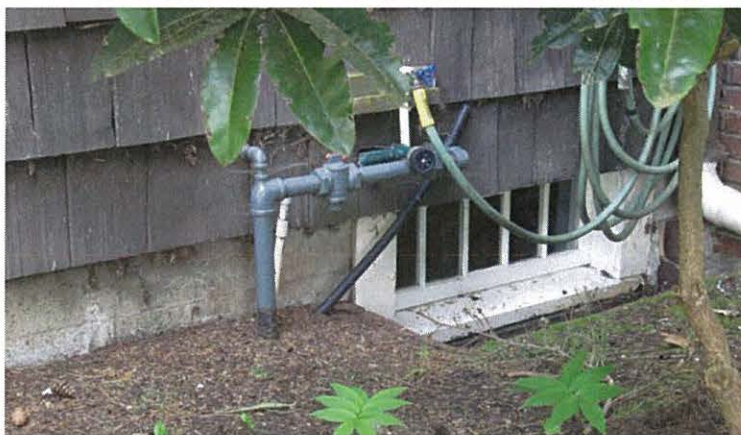
Basement level original windows and concrete foundation
