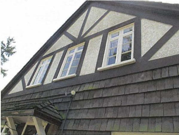
Windows in the gable end
