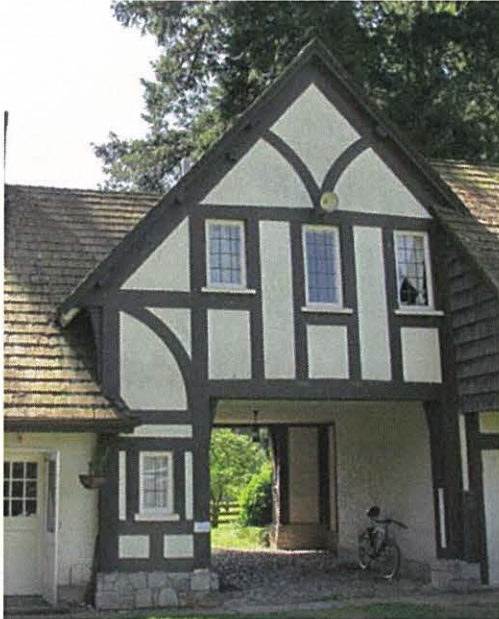
North elevation gable end: bargeboards, brackets and projected sills
