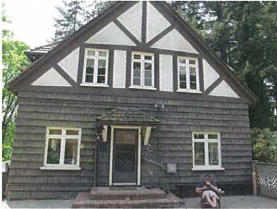
Side Entryway, north façade
