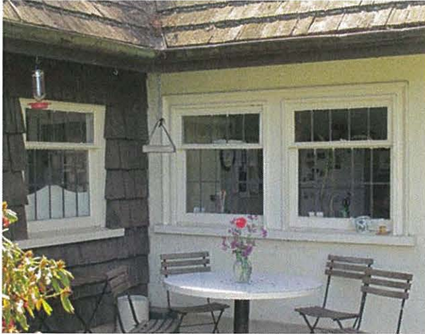
Original windows in the northeastern entryway area Broken window pane on south elevation
