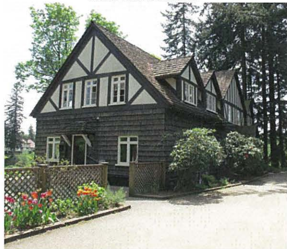
Roof structure from north
