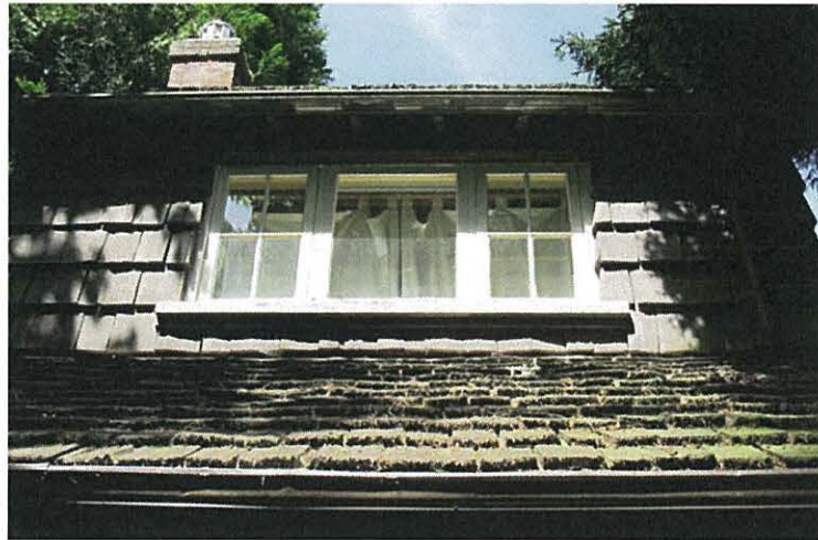
East elevation shed roof dormer with interior brick chimney on upper left
