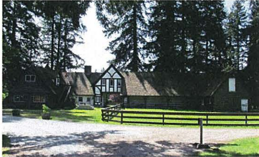
North (rear) facade
