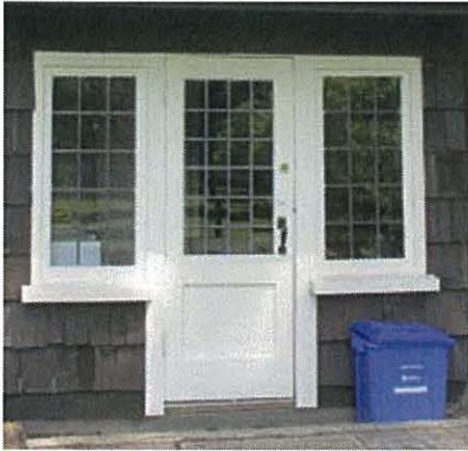
South elevation door assembly
