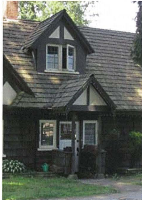
East elevation entryway
