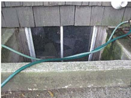
Replacement basement window
