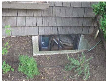
Replacement basement window
