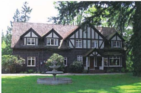
Front (west) facade
