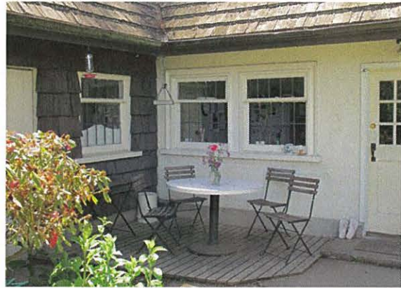
North elevation: stucco cladding at northeastern building entrance
