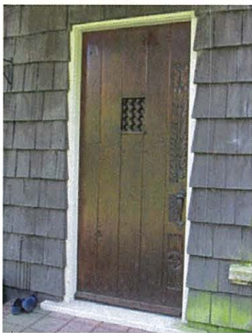
Original north elevation door
