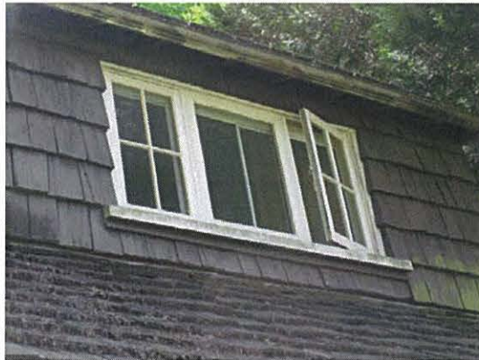
Original tripartite windows
