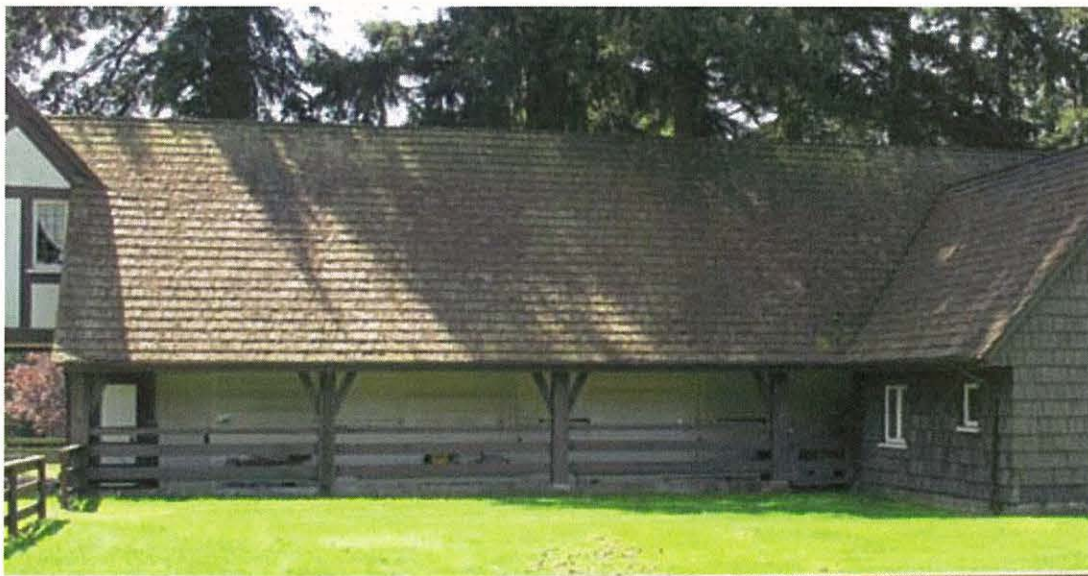
North elevation: columns supporting roof along former stables, along with fencing
