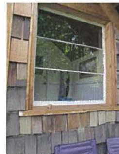
Replacement window of the addition
