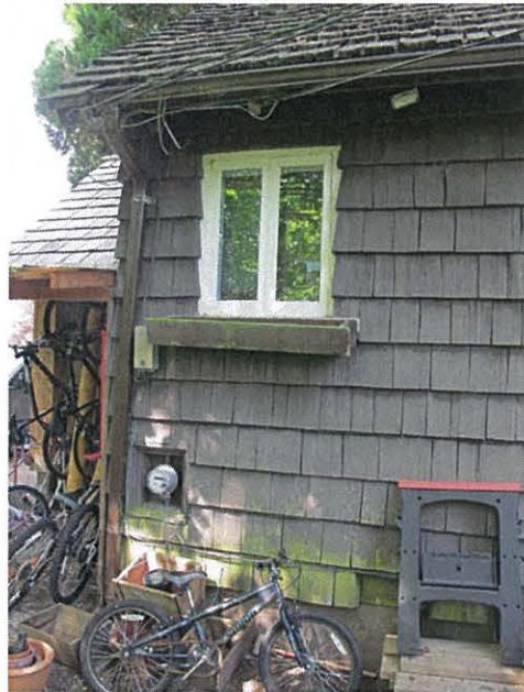
Original windows of the west façade
