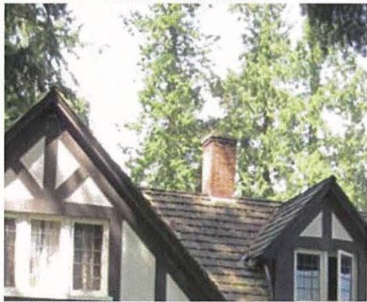
East elevation interior brick chimney
