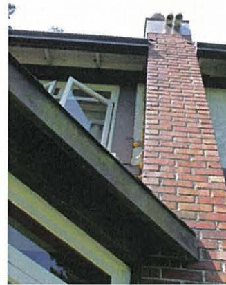
Chimney on east facade
