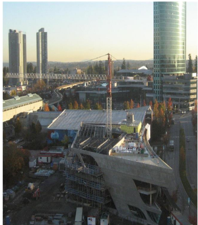
Surrey City Centre Library, under construction.
