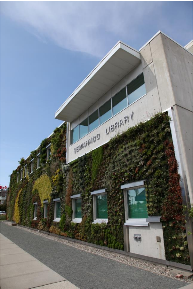
Living wall installed on Surrey’s Semiahmoo
