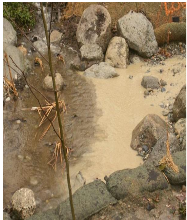
Sediment from poor site development practices.
